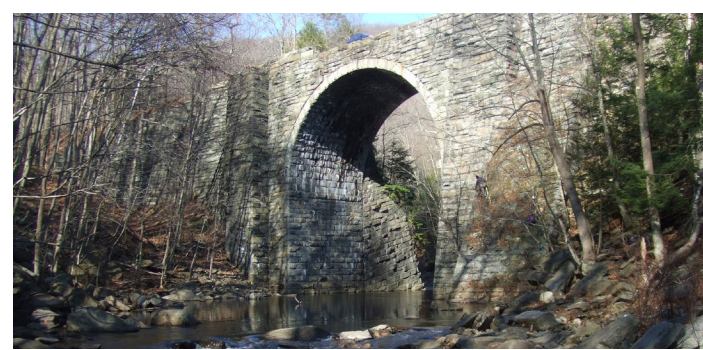
KEYSTONE ARCH BRIDGE
